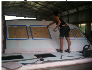
Central unit progresses - alongside hull panels
